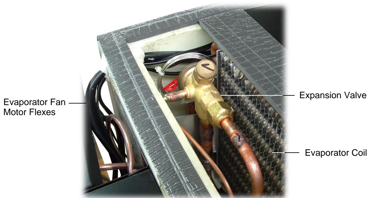
Figure 42: Expansion Valve
