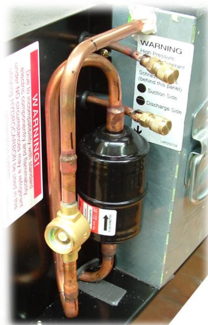
Figure 28: Liquid Line Sightglass
