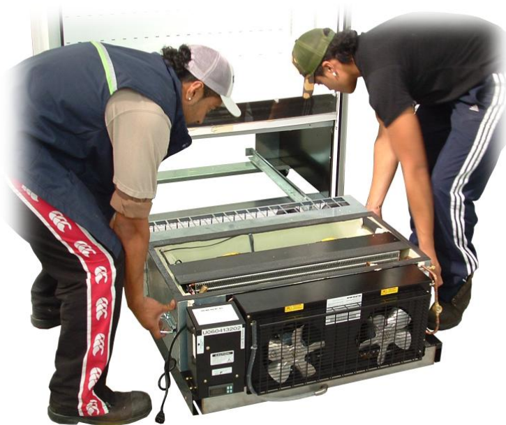
Figure 41: Refrigeration Unit (pulled out)
