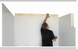
6. Slot the ceiling support brackets into the edges of the ceiling panel/s.
