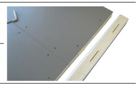
9. Silicone and slot a 2-way corner cap into each corner of the floor. The corner cap edges slide under the floor edge pieces for a tight fit.
