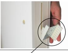
Lift the ceiling panel/s onto the room walls, hang using the ceiling supports and lock into place. If fitting multiple ceiling panels, fit the rear panel first and work forward.
